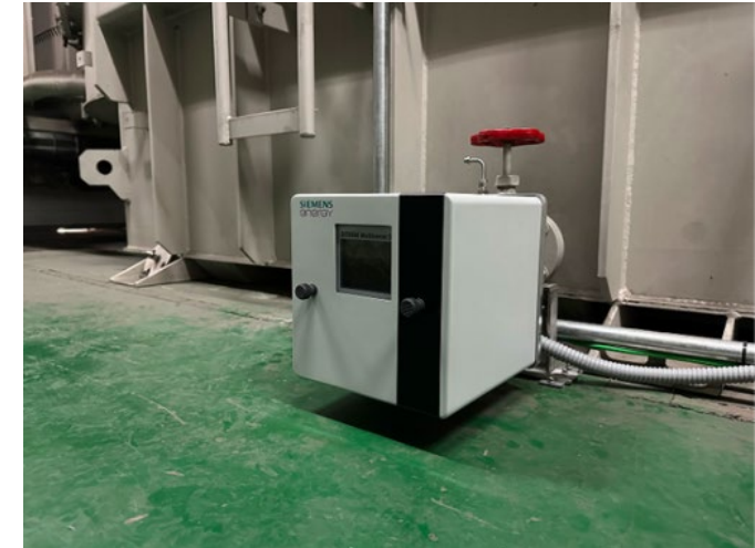
Installation Photo of DGA at KEPCO Substation
