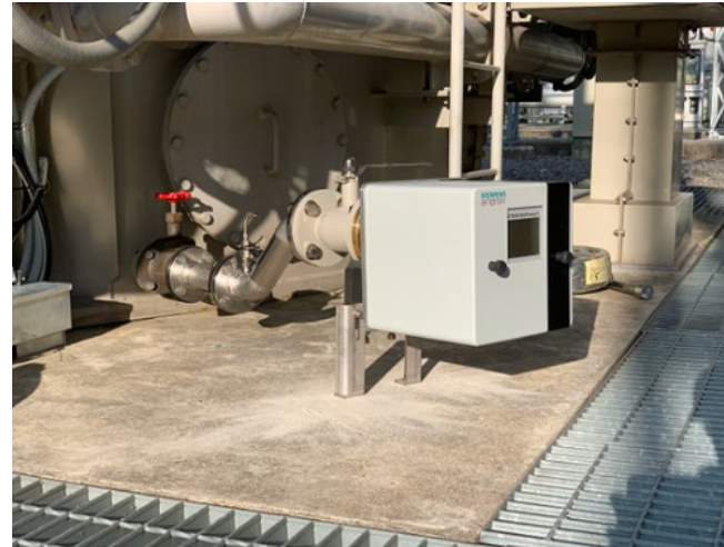
Installation Photo of DGA at KEPCO Substation
