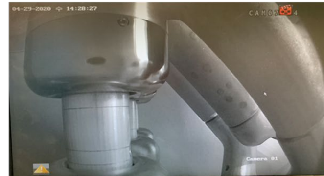
Visual Data of Disconnecting Switch Contact
